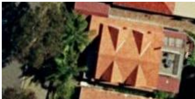
"Google maps" picture of our house roof
