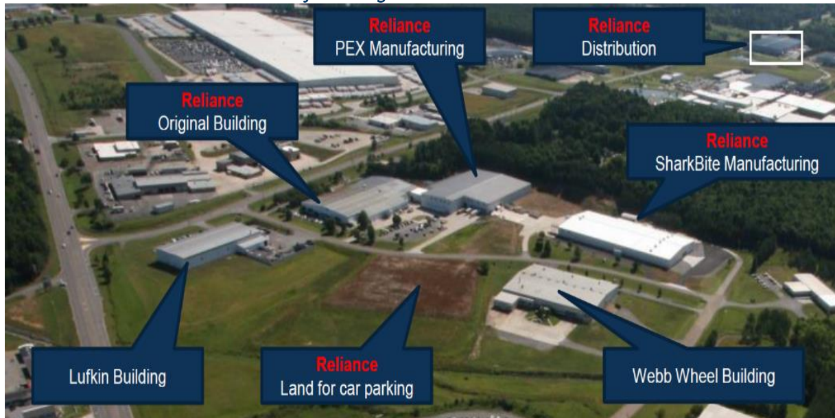
Photo 4: Reliance Alabama Manufacturing Facilities
