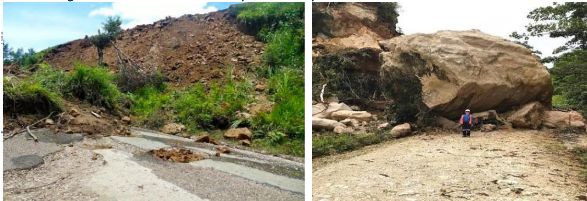
Photo 6: Highlands roads rendered impassable by landslides
