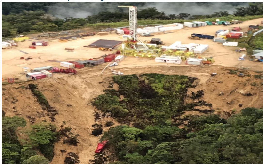
Photo 4: Moran well pad damage
