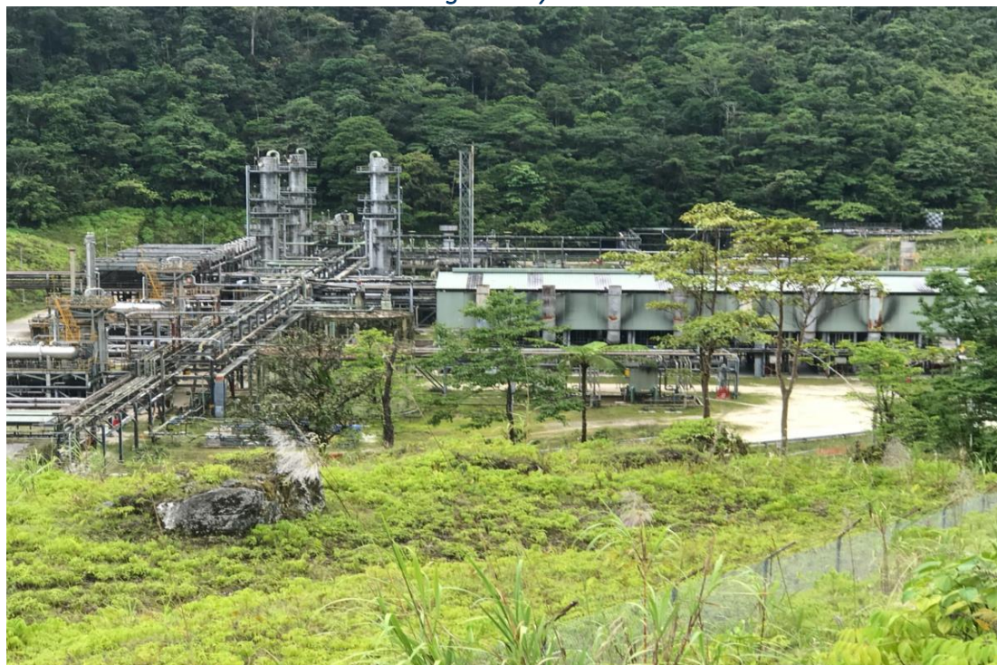
Photo 2: Oil Search Central Processing Facility
