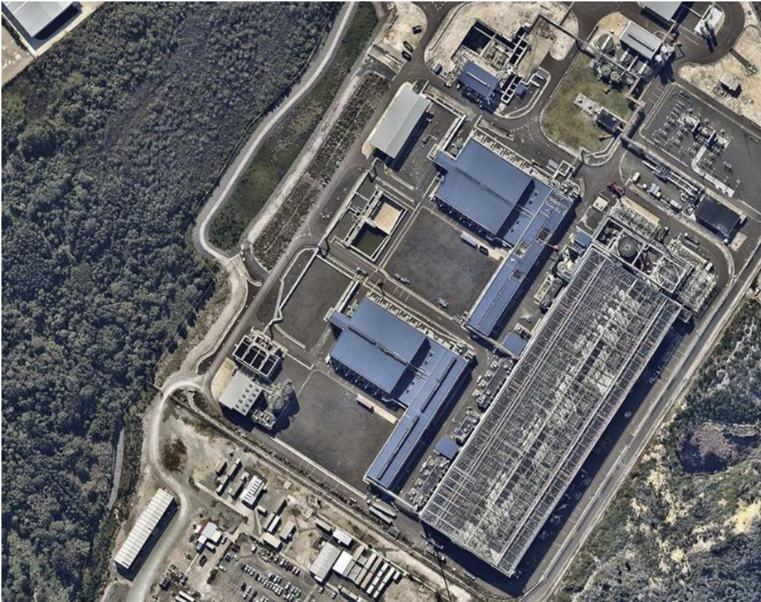
Photo 15: Desalination plant at Kurnell, NSW
