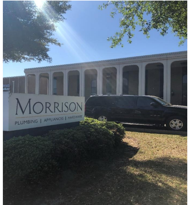
Photo 14: Morrison Lazybrook & Timbergrove (1)
