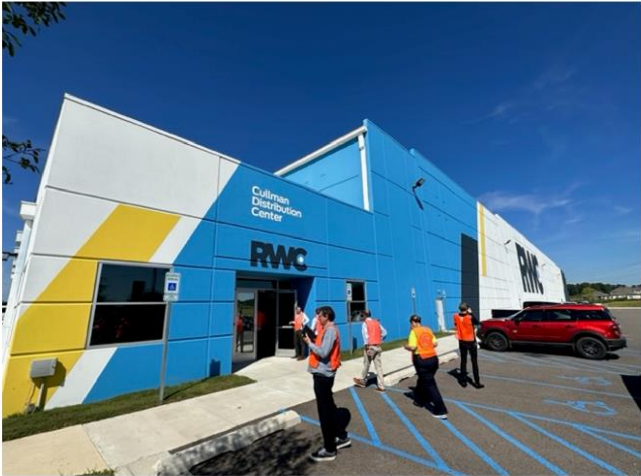
Photo 13: Reliance Worldwide Distribution Centre
